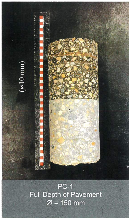
Photograph 1: Specimen from Ellice Avenue, Eastbound Curb Lane
